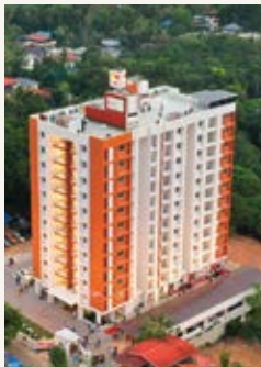
VARMA BOLGAN HEIGHTS COMPACT APARTMENTS CHOTTANIKARA, KOCCHI
