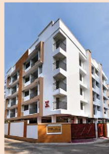
VARMA KOTTARAM LUXURY APARTMENTS TRIPUNITHURA
