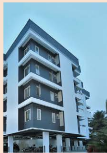
VARMA REGENT COMPACT APARTMENTS EDAPALLY
